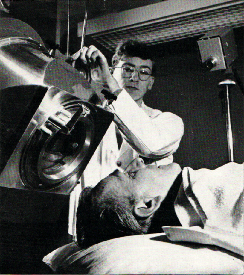
A Caesium Teletherapy Unit used in the treatment of cancers.
