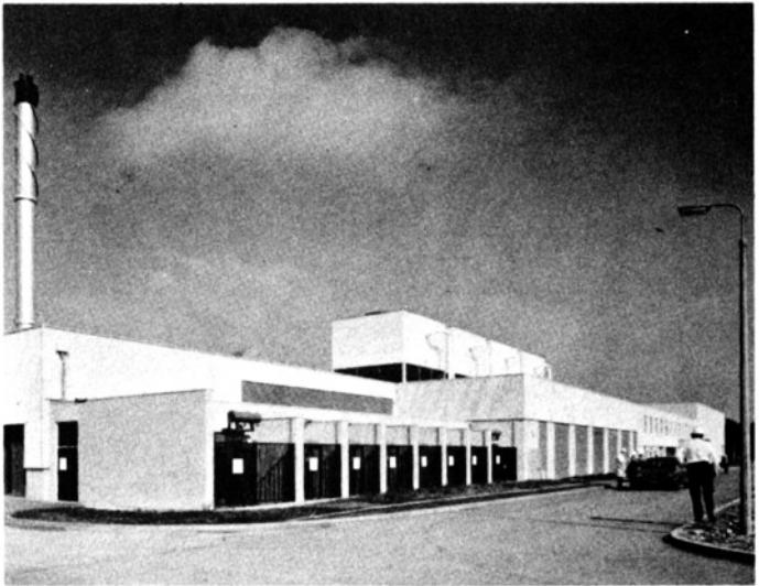
The new gas centrifuge plant at BNFL Capenhurst.
