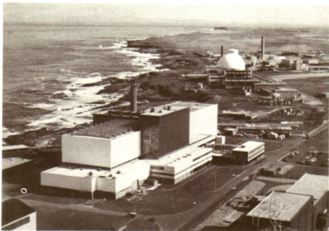
The 250 MW (e) Prototype Fast Reactor at Dounreay in Scotland.
