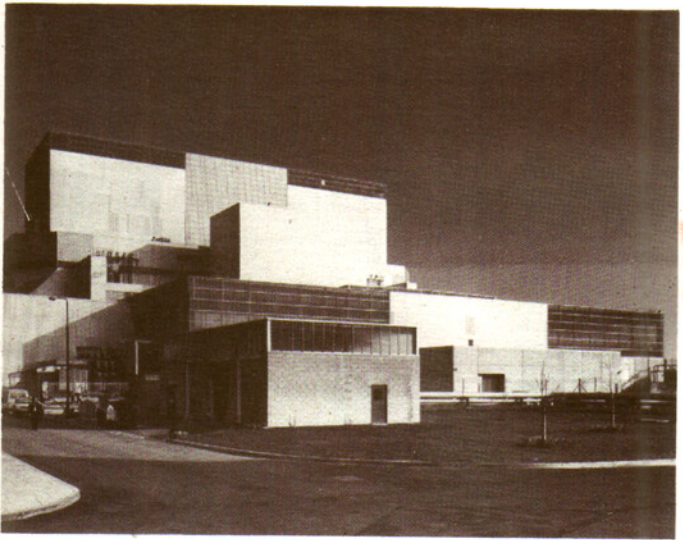
Hinkley Point B Advanced Gas-cooled Reactor power station in Somerset.
