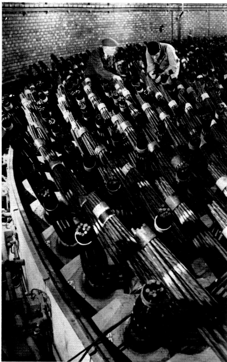
Fig. 3 Prestressing cables at Oldbury.
