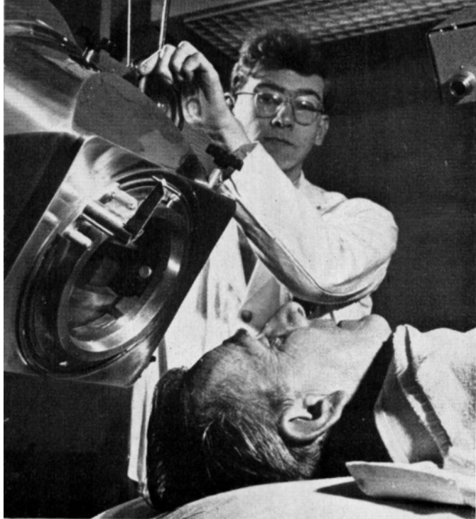
The Caesium 137 unit, installed at the Royal Marsden Hospital, Sutton, for the treatment of cancer.
